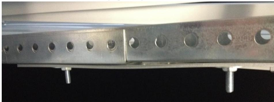
**Figure 5.** Reinforced Guide Rail
